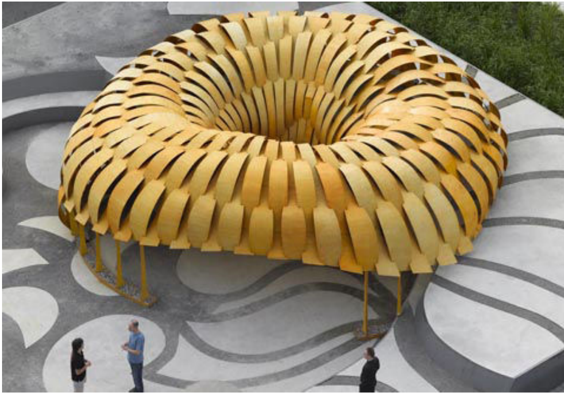
Figure 1.1.2 – The ICD/ITKE Research Pavilion 2010 made from thin, elastically bent plywood sheets
